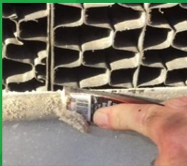
90 days into the demonstration, deposits inside the tubes and on the fill media did not increase after chemicals were reduced and the water concentration cycles were increased. Hard scale deposits began to soften and could be removed easily.
